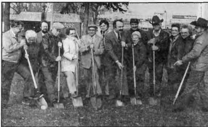
November 1984: Groundbreaking for construction of a museum headquarters building for the Iowa County Historical Society on North Bequette St., Dodgeville. Participants were, left to right: Frank Hess, Melva Phillips, Jim Jewell, Milo Mellum, Lyla Vinje, Ken Fox, John Swanson, Ron Dentinger, Bernard Sersch, Lucille Lauper, Vernon Bell, Marie Sersch, Charlene Murn, Jim Murn.
