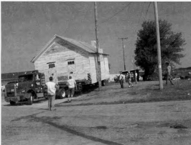
A close shave ... backing to the foundation site
