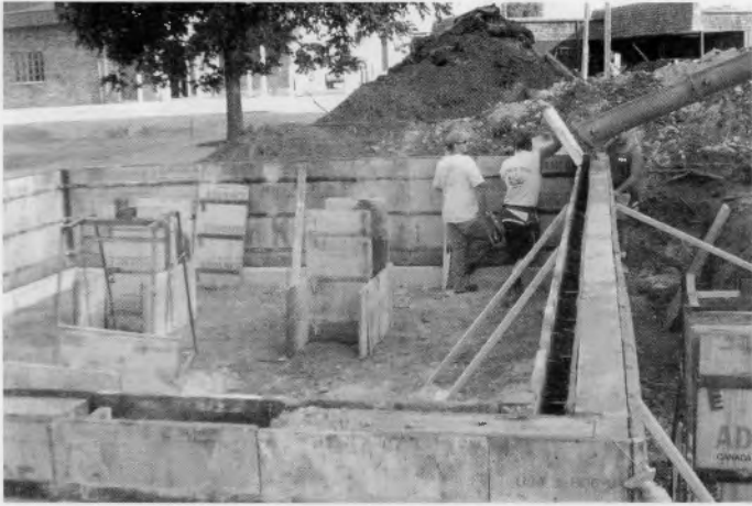
Pouring concrete at new Floyd School site
