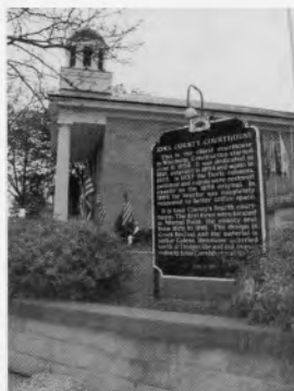
Courthouse at an angle
